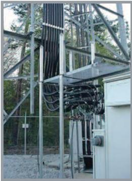
FIGURE 1: Wiring from tower antennas to base station
